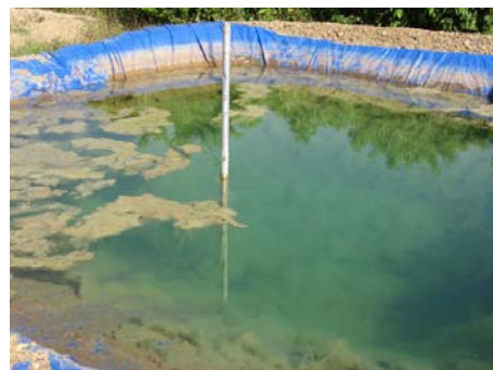
Figure 2. Silpaulin PVC Geomembrane tested in a pond at CARI Port Blair
