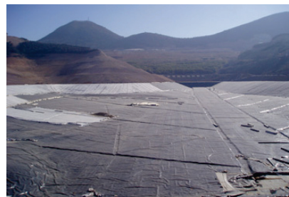
Figure 2. Construction of bottom geosynthetics system.
