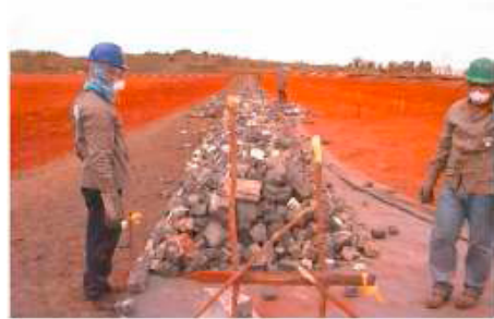
Figure 1. Construction of initial dike
