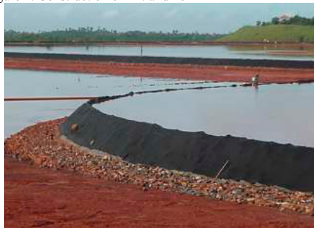
Figure 2. Operation of initial dike
