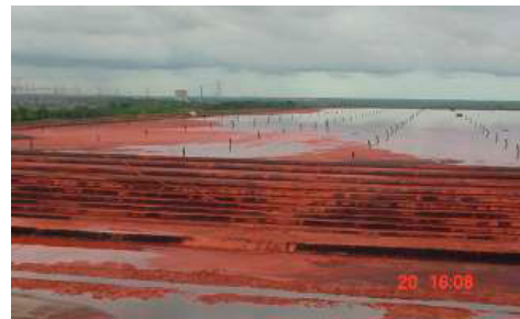
Figure 6. General view of stack
