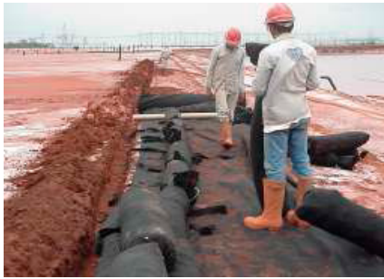
Figure 3. Assembly of dikes using geotextile tubes
