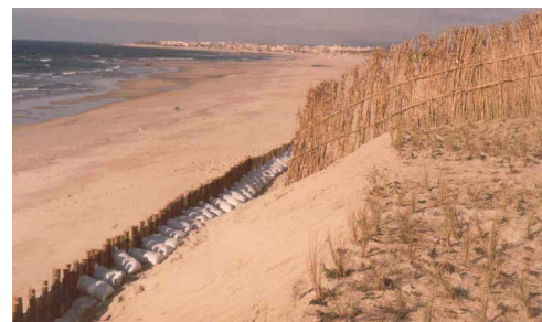
Figure 4 Dune consolidation with woodpiles and small bags full with sand, April 1999.
