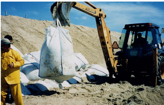
Figure 10 Geobag currently use in the strengthening of the dune of Estela.
