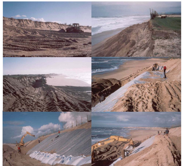
Figure 8 Construction sequence of the installation of the geotextile sand containers, December 2000.
