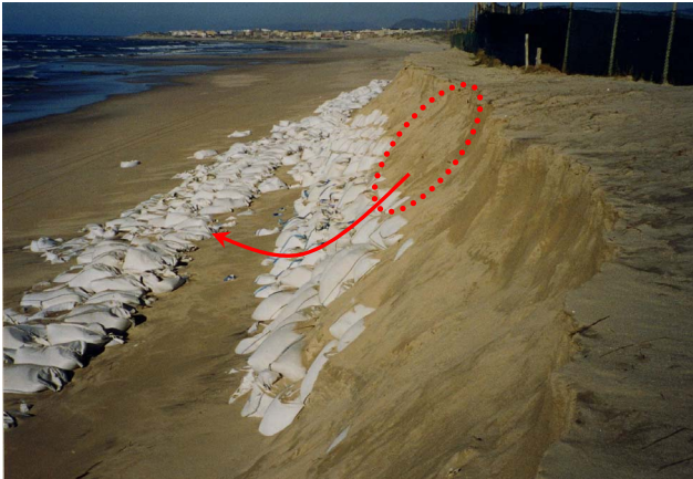
Figure 11 Probable mechanism of failure.
