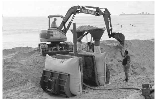
Figure 2 Filling geosynthetic containers (courtesy Geofilters Australia)
