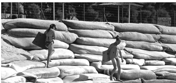
Figure 4 Geosynthetic containers for beach protection (WWF 2000)
