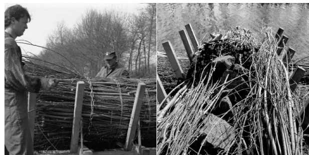
Figure 3 Preparing fascines for scour countermeasure
