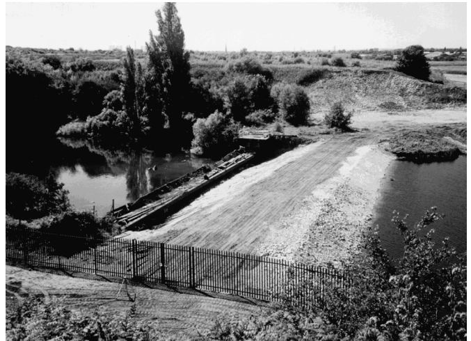
Photograph 6 Completed eastern embankment.
