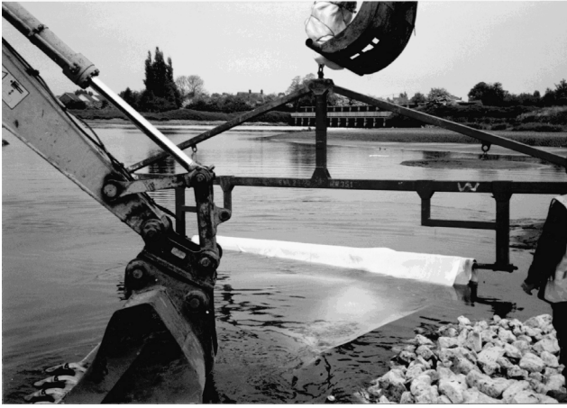
Photograph 1 Eastern Closure Placing Basal Geomat
