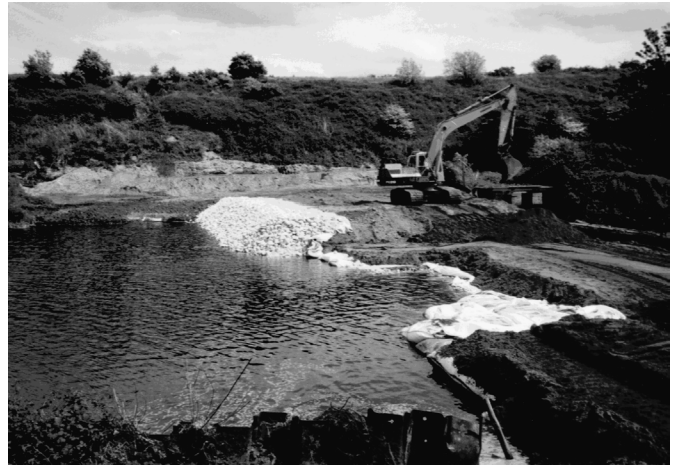
Photograph 5 Construction above water level.
