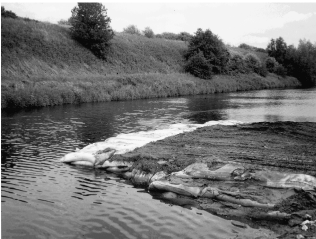
Photograph 4 Southern Closure – Geobag Base with Sand Protection
