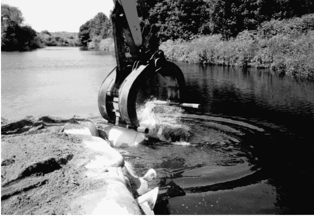
Photograph 3 Southern Closure Placing Geobag Below Water
