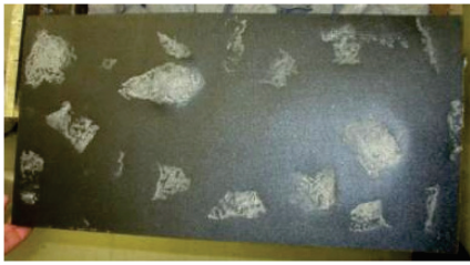
Figure 8. Condition of TLS surface after loading test (No. B-1).
