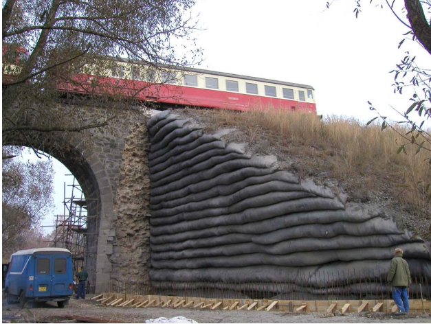
Figure 9 Reinforced soil wall after the stonewall removal
