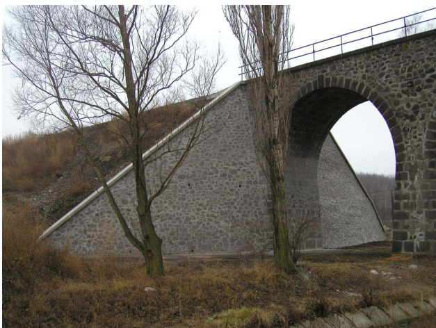
Figure 10 Reconstructed bridge and the embankment
