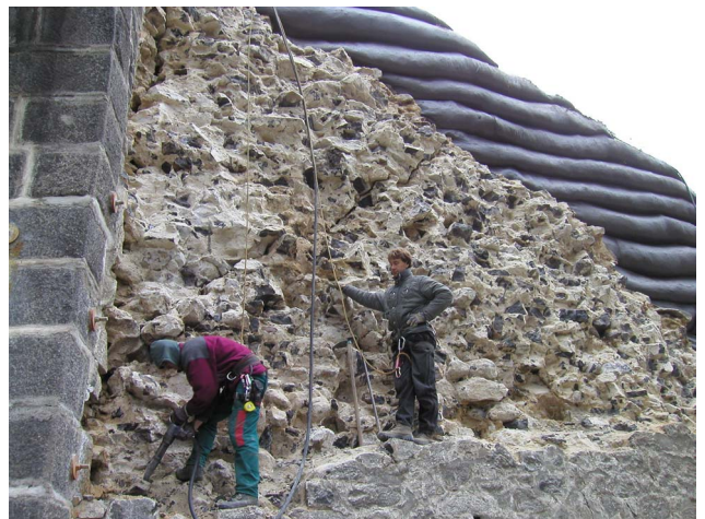
Figure 8 Demolishing of the upper part of the stone wing wall
