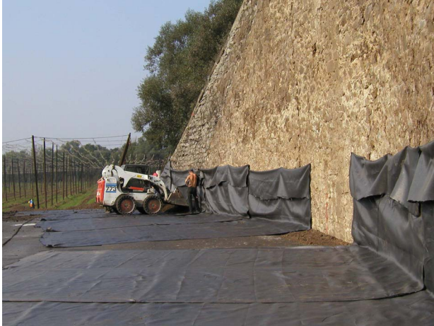
Figure 5 Laying geotextile reinforcement on the compacted soil
