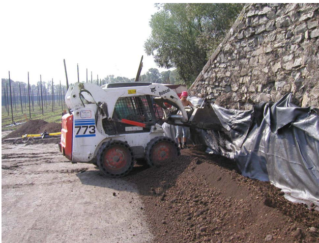
Figure 6 Placing lightweight ceramic aggregate on the geotextile near the abutment
