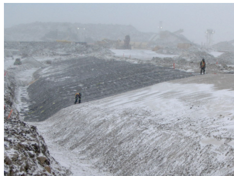
Photo 4. Liner installation.
