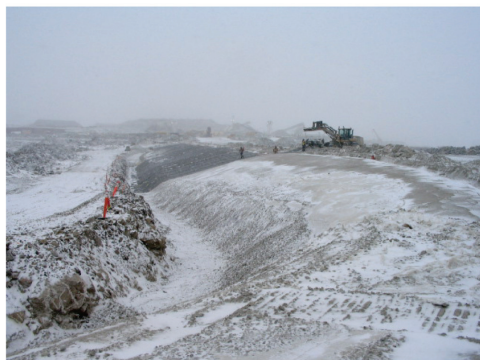
Photo 3. Bottom of trench.
