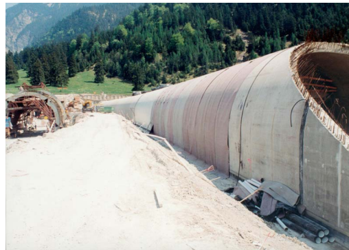
Figure 2 Vault tunnel with geomembrane sealing via cut-and-cover construction method during construction
