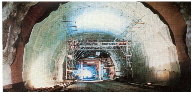
Figure 1 Trenchless two-shell tunnel with geomembrane sealing during construction
