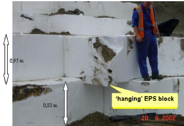
Figure 11 After excavation visible overloaded and permanently deformed (compressed) EPS-blocks on the front (southern) side of light-weight approach road structure along axis M100
