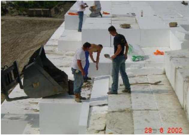
Figure 12 Improvised levelling of asymmetrical deformation in the cross section on axis M100 by means of too thin EPS-blocks which as such might not be used at all according Dutch standard
