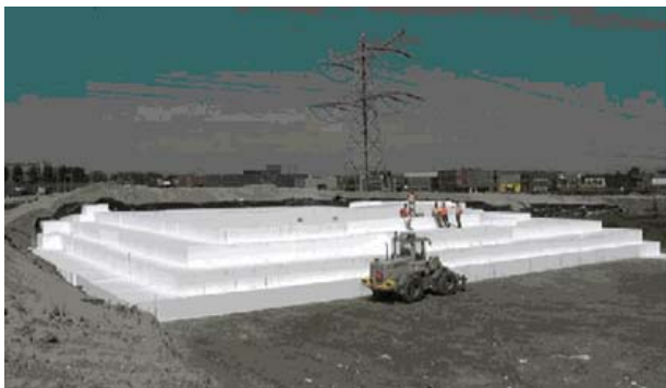
Figure 2 Partly covered EPS-blocks of the monitored approach road on the north side of the Sliedrecht-East junction
