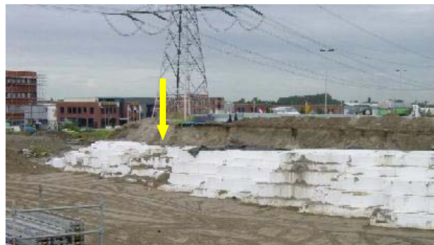
Figure 12 Asymmetrical deformation in the cross section of light-weight road embankment due to not taking into account preload history (1999-2001) in the northern quadrant of the Slidrecht-East junction
