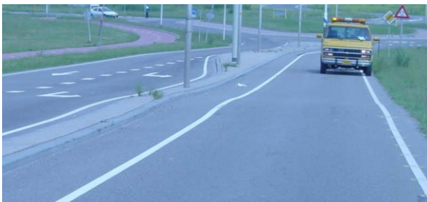
Figure 13 'Threshold' arisen between on road founded on piles and light-weight road parts along axis MR100 due to settlement differences
