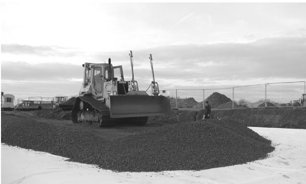
Figure 14 Placing of drainage gravel on geotextile protected geomembrane
