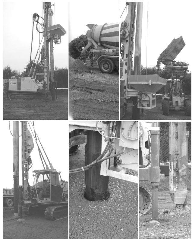
Figure 12 Equipment and procedure to install vibro concrete columns
