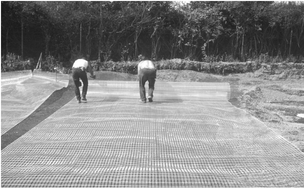
Figure 13 Laying of geogrids
