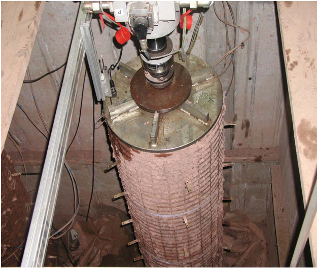
Figure 3 Head area of the geogrid- wrapped mineral-material column
