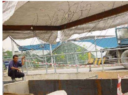
Figure 4 – Geotextile with strain gauges being installed in the pit
