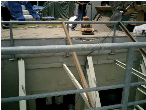
Figure 2 – Final embankment of experiment 2 before traffic tests
