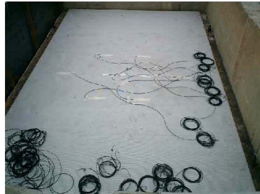
Figure 3 – Layers of geotextile crossed and fixed on a steel frame
