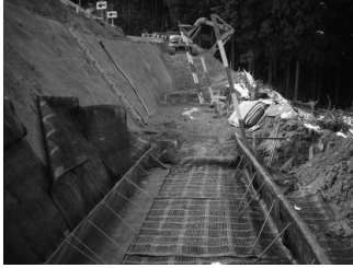
Photograph 3. Install the geogrid
