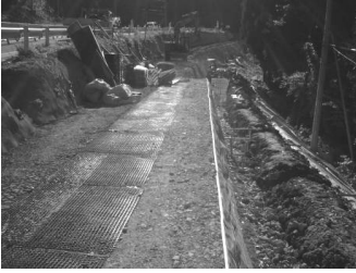
Photograph 4. Wrap the geogrid
