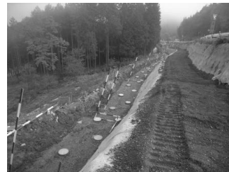
Photograph 2. Install the pile
