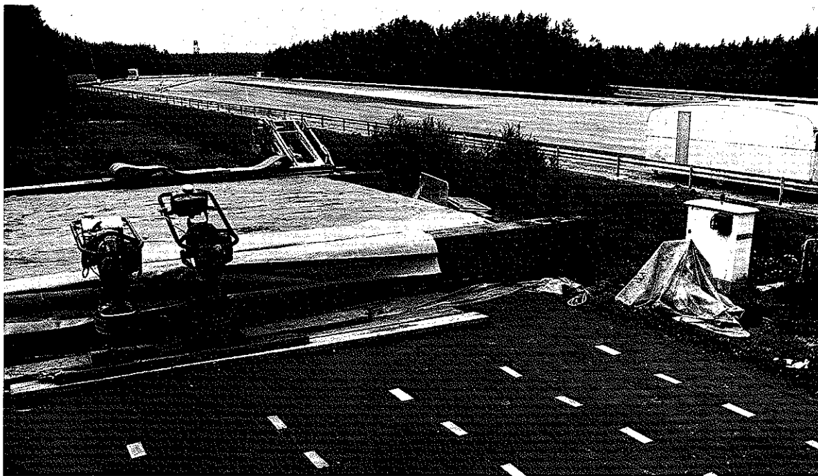
PLATE 1. LAYOUT OF SPECIMENS IN THE CLAY EMBANKMENT ALSO SHOWING THE COMPLETED SAND EMBANKMENT AND THE COMPACTION PLANT USED.
