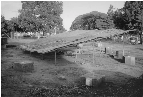
Figure 1. Panel with geomembranes exposed to weathering degradation
