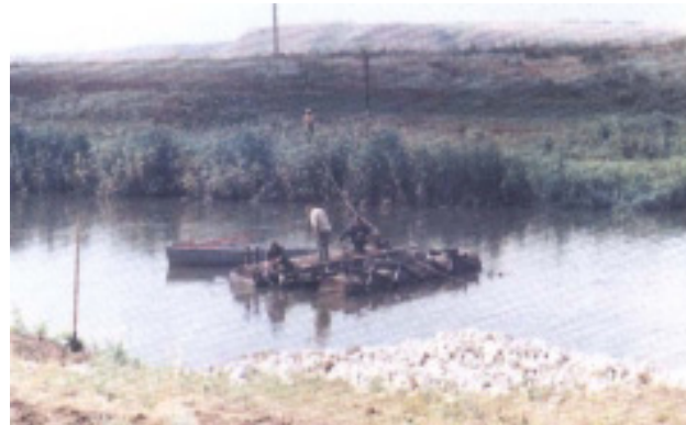
Figure 2. Laying of AEC Cover in river-bed section area of crossing.
