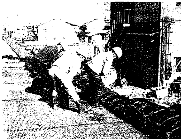
Plate 3 Piling up gabions
