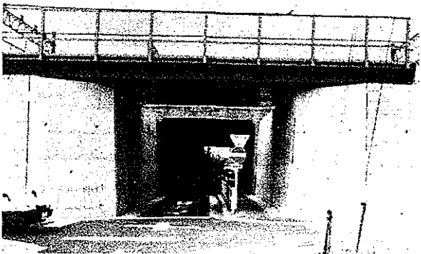
Plate 6 After the construction of the permanent over-road bridge
