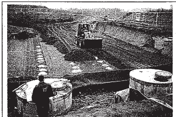
Figure 4. The first geogrid layer with installed measurement devices
