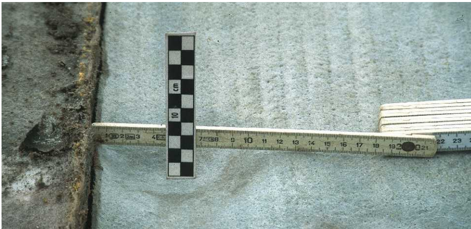
Figure 1. Bentonite mat with indentation caused by riprap
