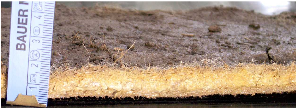
Figure 3. Section through a sample of a bentonite mat taken from the Kinzig Dike
