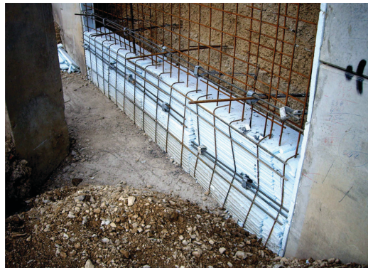
Figure 6. Repairing jobs. Elastic joint of expanded polystyrene placed at the footing.
