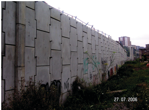
Figure 5. Huge settlements (0.5 m–0.75 m) suffered along the wall's facing with no cracked panels reported at all. See the horizontal joint's deflection.
