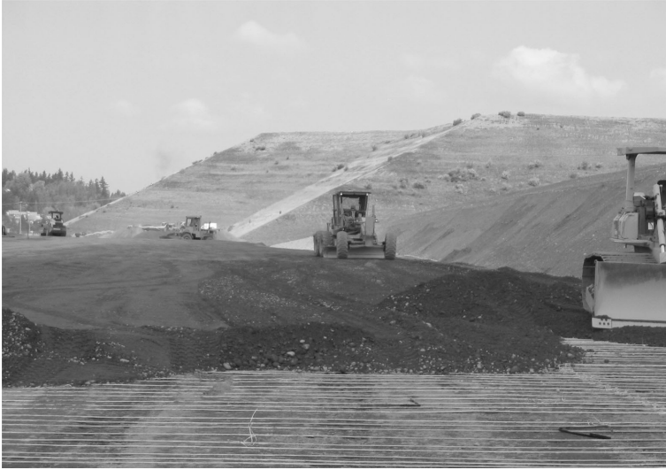
Figure 3. Reinforcing strip placement.
