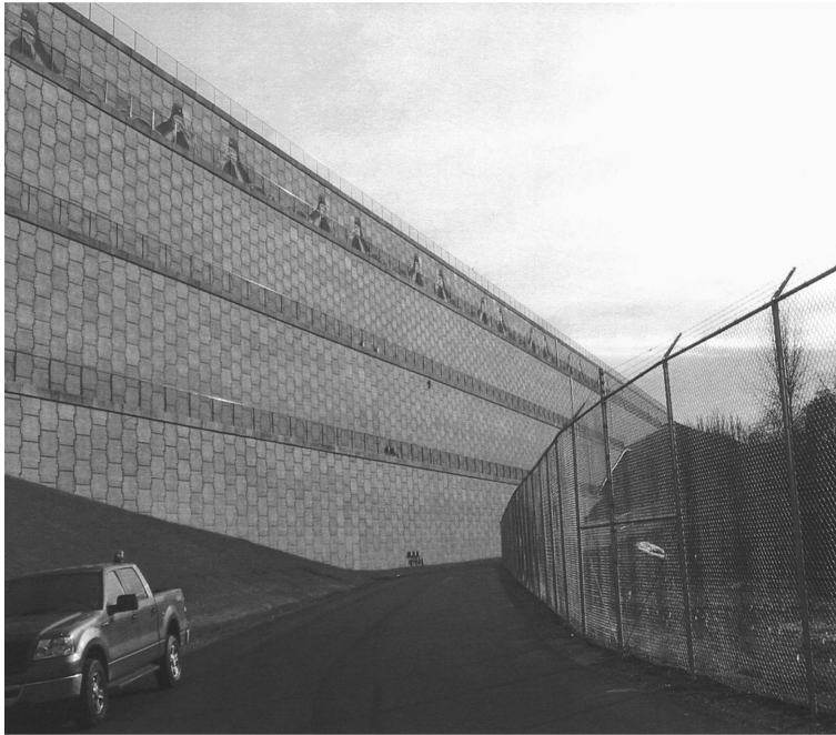
Figure 5. View of completed four tier Reinforced Earth wall.
