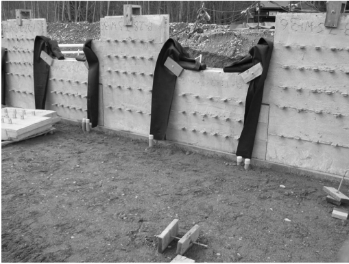
Figure 2. Tie strips ready to receive reinforcing strips in lower tier panels.
