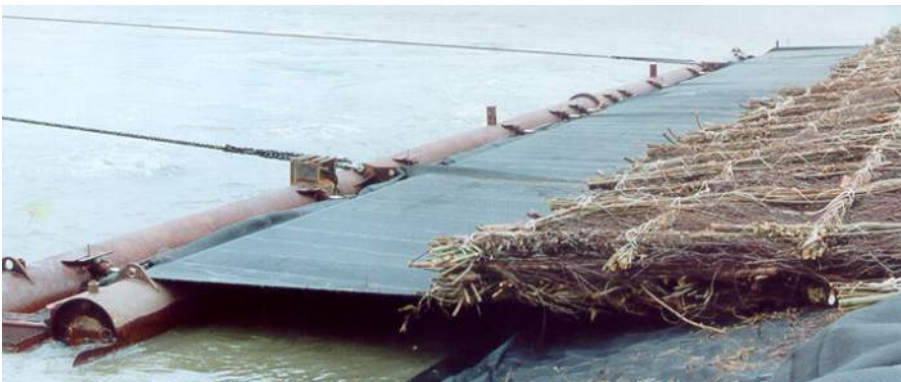
Figure 2: Fascine mattress attached to the sinker tube
