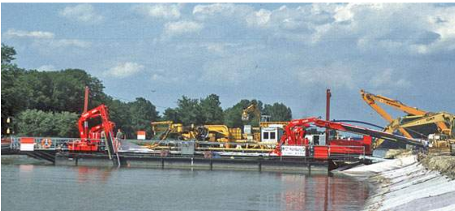
Figure 5: Geotextile installation by unrolling
