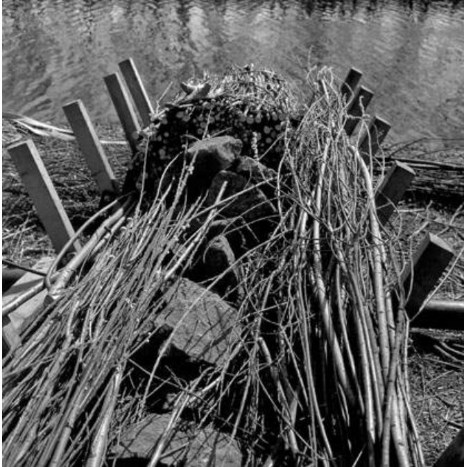
Figure 3: Preparing a large Fascine with riprap core
