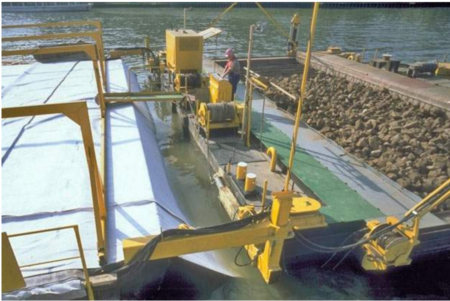
Figure 4: Geotextile installation pontoon and stone dumping unit
