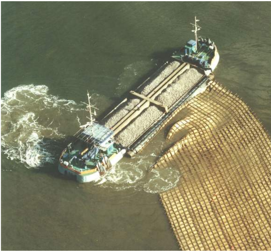
Figure 1: Pulling a fascine mattress to the installation site
