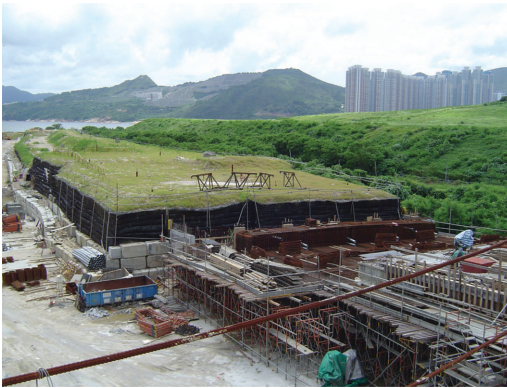
Photo 4. End view of reinforced surcharge block (Tseung Kwan O).
