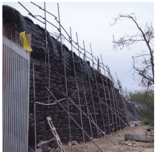
Photo 6. Surcharge embankment at site boundary (Tseung Kwan O).
