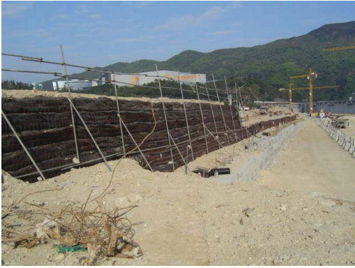
Photo 7. Surcharge embankment under construction (Tseung Kwan O).
