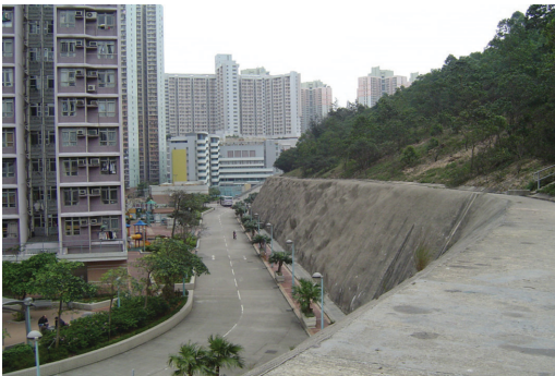
Photo 3. Estate road occupies early haul road (Po Tat Estate).
