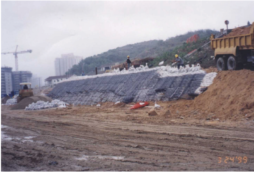
Photo 2. Construction of haul road (Po Tat Estate).
