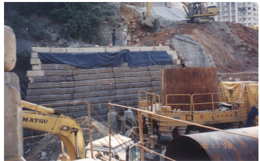
Photo 1. Temporary work platform with access ramp behind (Belcher Garden).
