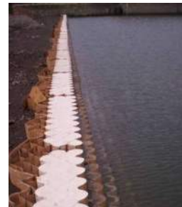
Figure 4. Isometric view of Geocell Connection Figure 5. Geocell armour during construction
