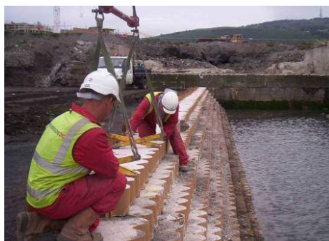
Figure 7: Positioning Geocell Armour Layer
