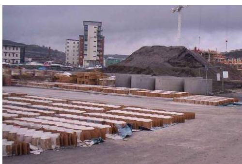
Figure 6. Precast Geocell Armour Layer
