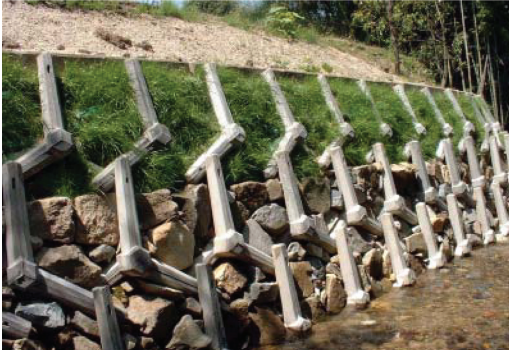
Figure 2. Configuration of proposed block wall using traditional stone masonry for river revetment in February 2003.
