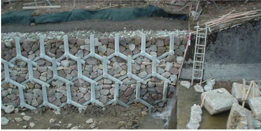
Figure 9. Reconstruction of river revetment after flood disaster.
