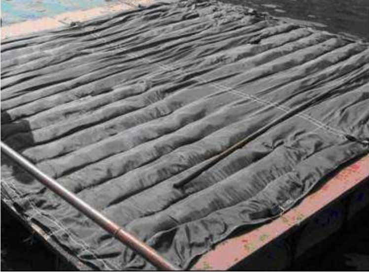
Figure 11. Sand mattress on the barge
