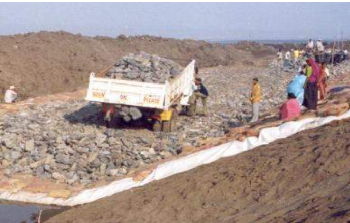
Figure 8. Rehabilitation of Sea wall at Moti-danti, Gujarat, India
