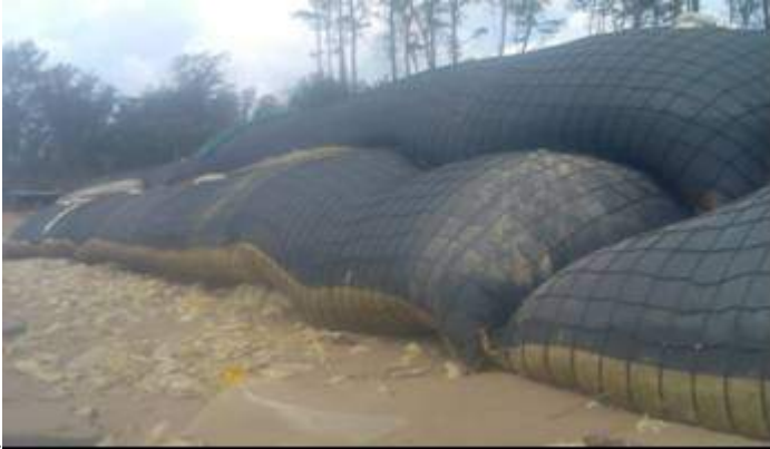
Figure 6. Completed protection coastal work at Shankarpur, West Bengal state, India
