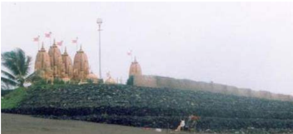
Figure 3. Sea wall at Tithal to protect Swaminarayan temple
