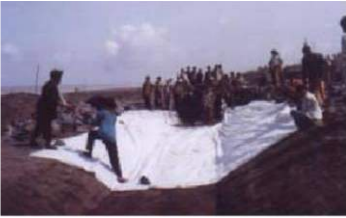
Figure 7. Installation of geotextile under gabion wall
