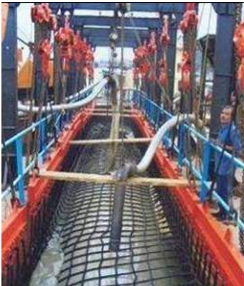
Figure 1. Filled geotextile tube in the splitting barge
