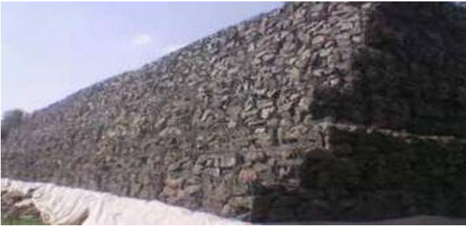
Figure 10. Geotextile under the Gabion wall
