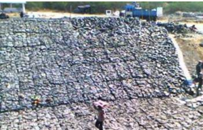
Figure 9. Bank protection work for Tapi River
