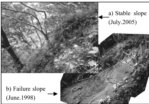
Figure 9. Izuinotori slope before and after rein-forcing by Non-frame.
