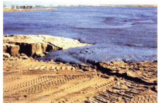
Photo 1. View of dredged clayey soil blow-out.
