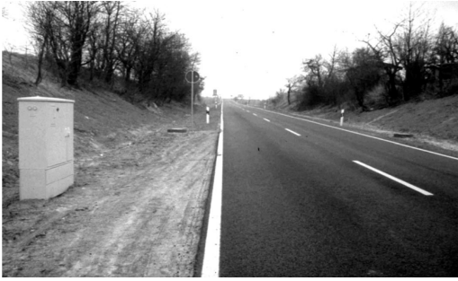
Figure 6. The B180 after completion: the carriageway, two of the control chambers and the warning system automatic switching cabinet.
