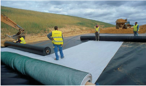
Photo 4. Installation of the reinforcement composite between 2 layers of geomembranes.
