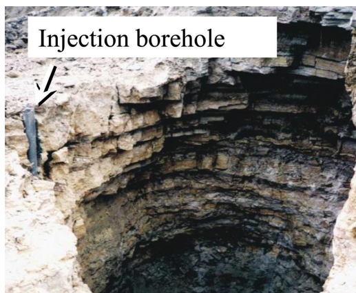
Photo 2. Cavity discovered during the construction close to an injection borehole.
