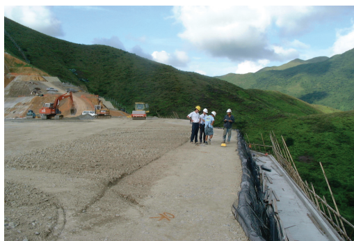
Figure 4. Compaction and testing of fill material.
