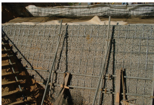
Figure 2. Completed gravel facing.
