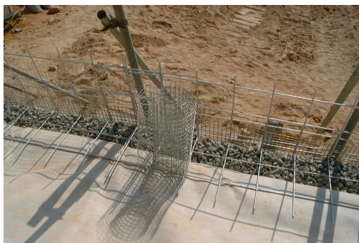
Figure 1. Gravel facing for fire resistance.
