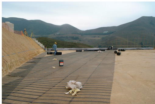
Figure 3. Placing geogrids on a curved alignment.
