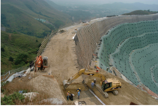
Figure 5. The embankment nearing completion.
