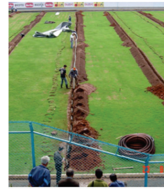
Photo 2. Insert of the geocomposite drain and placement of the withdrawn soil.
