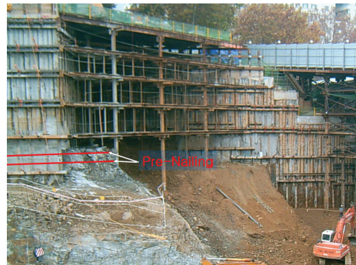
Photo 2. Construction of pre-soil nailing.
