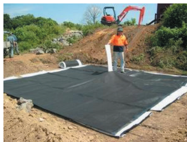
Photo 1. “Layflat” empty geotextile tube with inlet sleeve.
