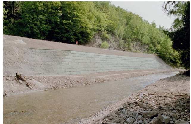
Figure 12 Facing of geogrid reinforced railway embankment
