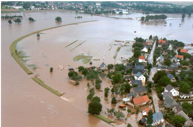
Figure 1 More than 100 dyke failures and floodings in 2002
