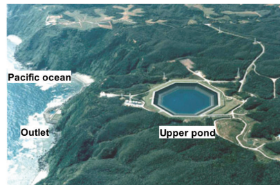
Figure 1. General view of the seawater pumped storage power plant.
