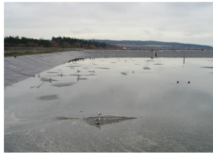
Figure 2. Emerging areas of geomembrane upon initial filling of the lagoon.
