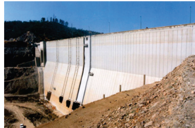
Figure 2. Pracana dam, Portugal 1992: PVC geomembrane.
