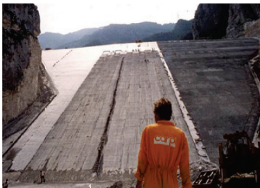
Figure 1. Bovilla fill dam, Albania 1996: PVC geomembrane.
