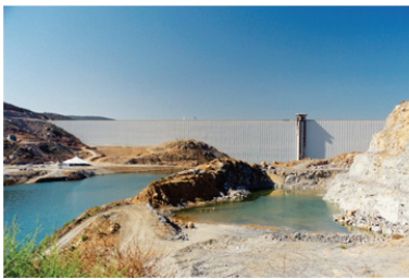
Figure 3. Olivenhain RCC dam, USA 2003: PVC geomembrane.
