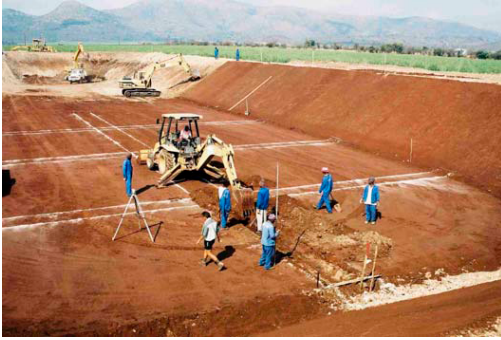
Plate 2: Bulk earthworks
