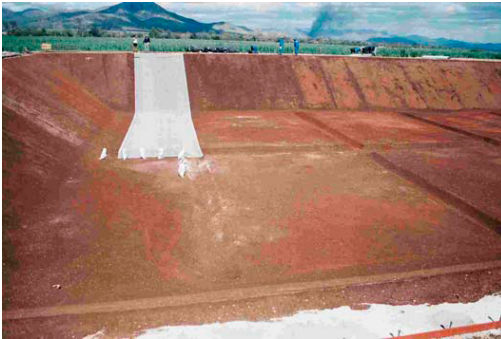
Plate 3: First installation of GCL on clay protection layer
