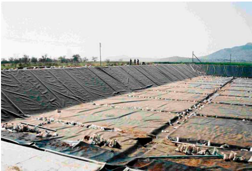
Plate 4: Installation of HDPE liner
