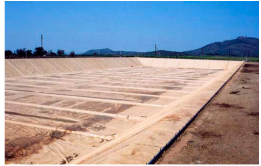
Plate 5: Installation of fPP-R cover
