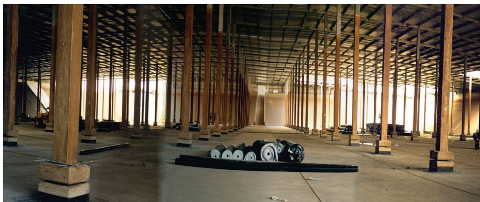
Figure 1. A typical view of Tamworth Hill Reservoir interior.
