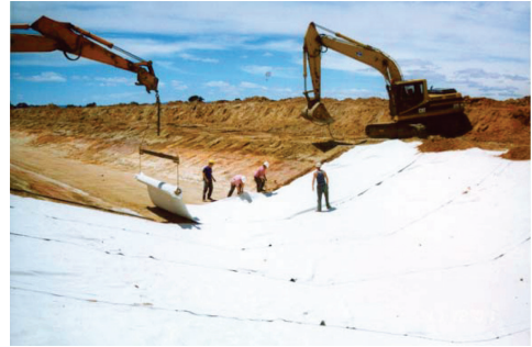
Figure 3. GCL installation.
