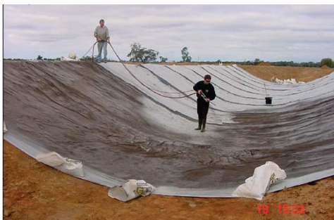
Figure 6. Rubberised bitumen emulsion.
