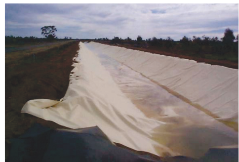
Figure 4. Reinforced PP a1.1 mm.
