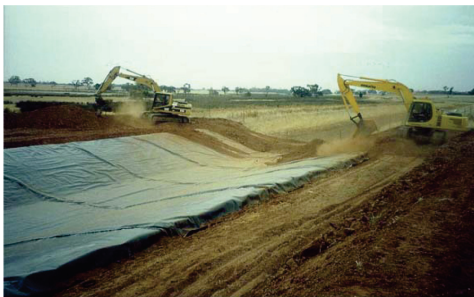
Figure 2. Soil cover installation over 0.75 mm HDPE.
