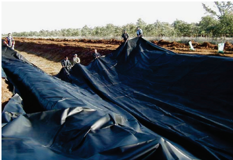
Figure 5. Unreinforced PP 0.75 mm (Note large crew size).
