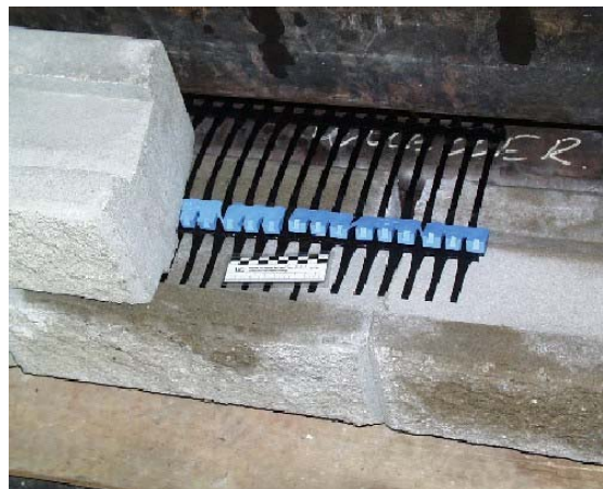
Figure 3: Photograph of the application of geogrid with connector (by tBU)
