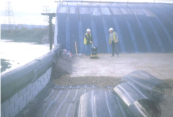
Figure 8: Photograph of the construction of the bridge in U.K.
