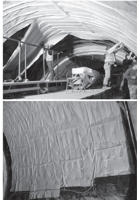
Figure 9. Installation of energy geotextiles at the testing plant "LT22 – Bierhäuselberg".
