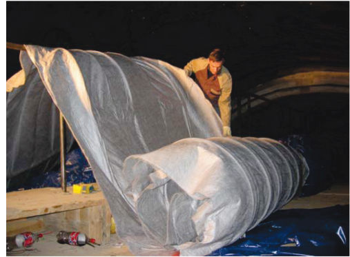
Figure 2. Unrolling of an energy geotextile.
