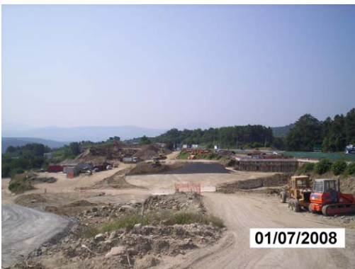
Fig. 14 – Construction of the base reinforced embankment
