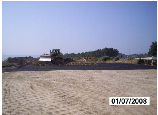
Fig. 16 – Geogrid installation for the base reinforced embankment
