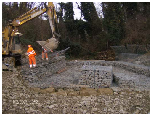
Fig. 10 – Filling gabions of the channels
