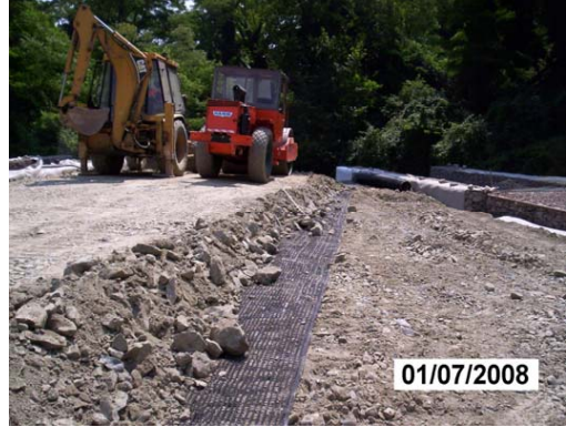
Fig. 9 – Fill compaction over geogrid reinforcement
