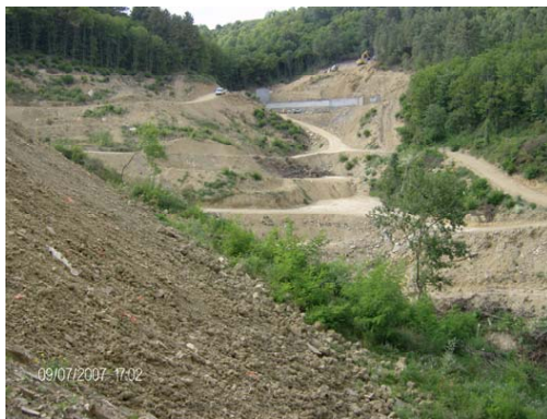
Fig. 7 – The valley before embankment construction
