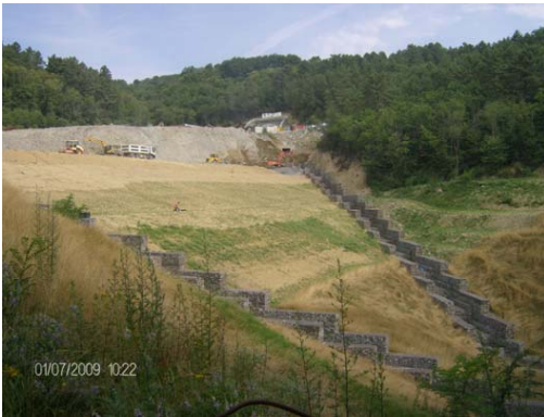
Fig. 13 – The reinforced embankment and the gabion channel almost completed
