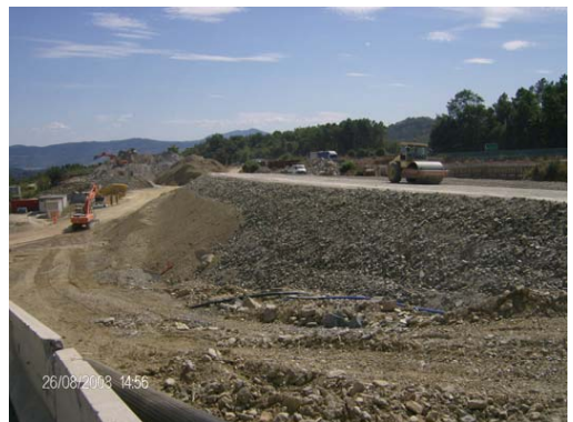
Fig. 17 – The base reinforced embankment near completion
