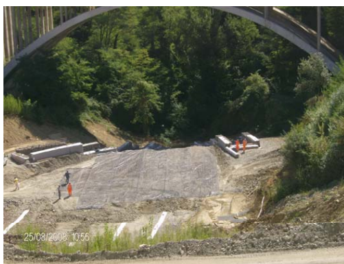
Fig. 8 – Laying the first geogrid layer
