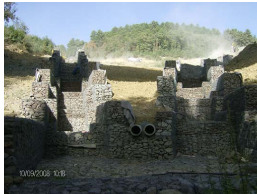
Fig. 11 – The gabion channels seen from the toe
