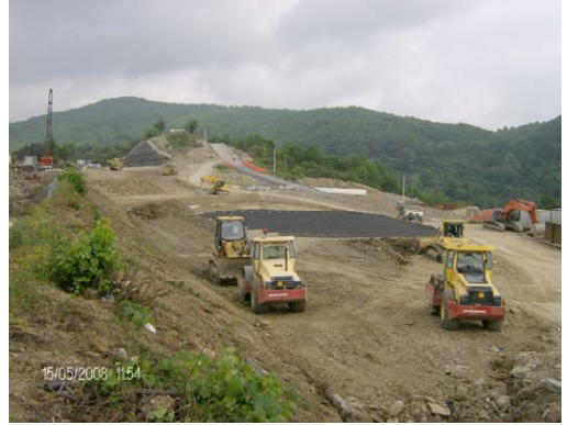
Fig. 15 – Construction of the base reinforced embankment
