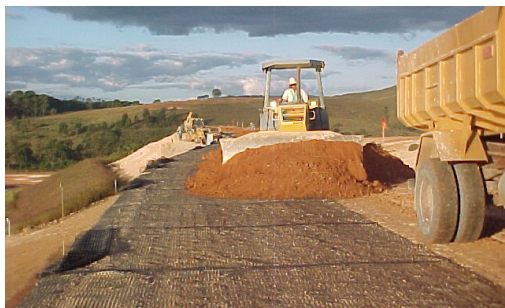
Figure 2. Construction of the geogrid reinforced wall
