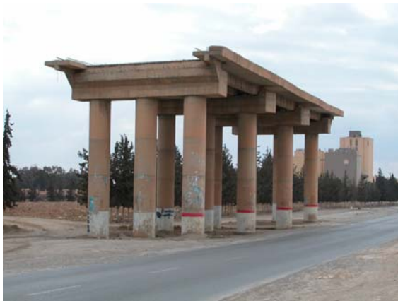
Figure 1. View of the unfinished bridge structure.
