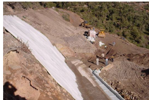
Figure 10. View of the geocomposite drain and drain trench.
