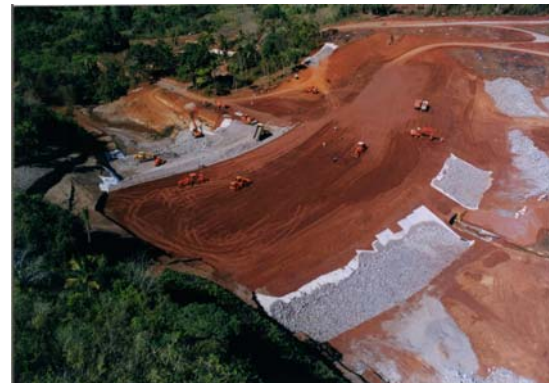
Figure 29. Top view of the dam during construction (filtration geotextile in white)
