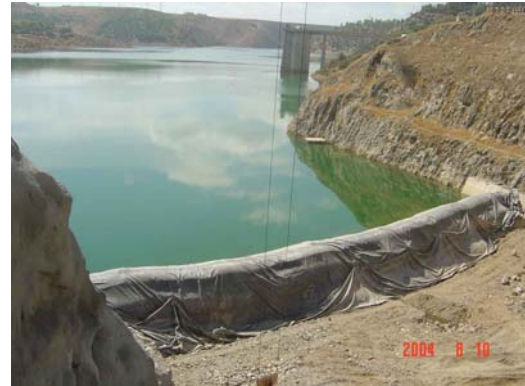
Figure 35. View of the dam with the geotextile tubes in place
