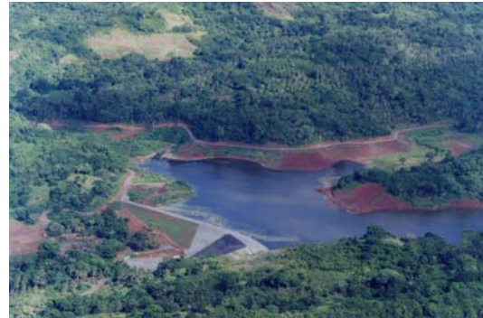
Figure 31. View of the completed dam.
