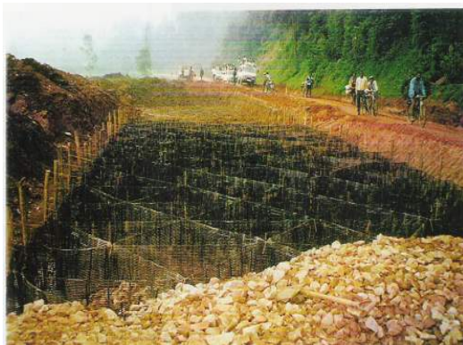
Figure 22. Construction of Geocell foundation mattress
