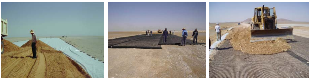
Figure 17. Installation of filtration geotextile, fill material and geogrid.
