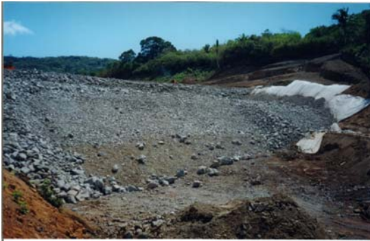
Figure 30. Drainage blanket with stone and filtration geotextile
