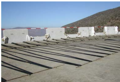
Figure 13. View of the geostrap reinforcement
