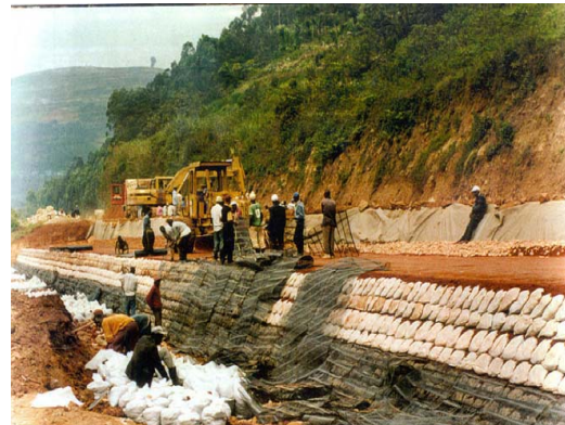
Figure 23. Construction of steep embankment slope.
