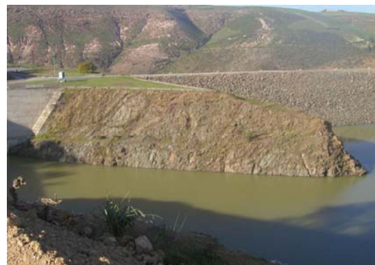
Figure 33. Overview of the site where the systems are being installed in the water. The walls have a height of around 50 meters.
