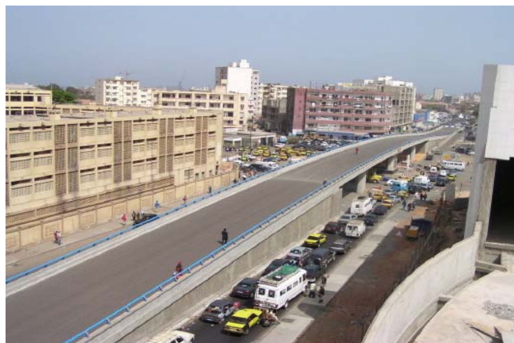
Figure 6. View of the completed structure.
