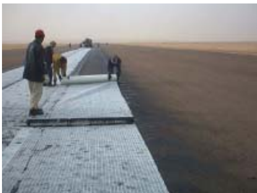
Figure 26. Installation of geogrid
