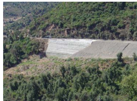
Figure 12. View of the completed wrap around geotextile wall.
