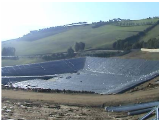
Figure 37. Geomembrane liner for a new cell
