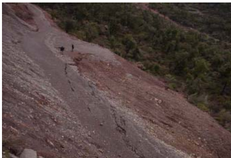
Figure 9. Longitudinal cracks caused by soil surcharge
