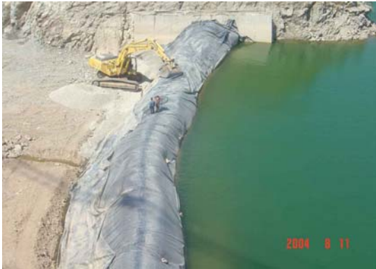
Figure 34. Dam in place and covered with the geomembrane.
