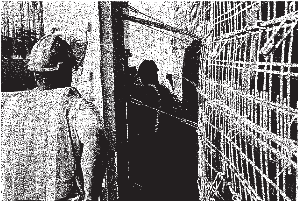
Figure 2. Connection of precast panels to wirewall.
