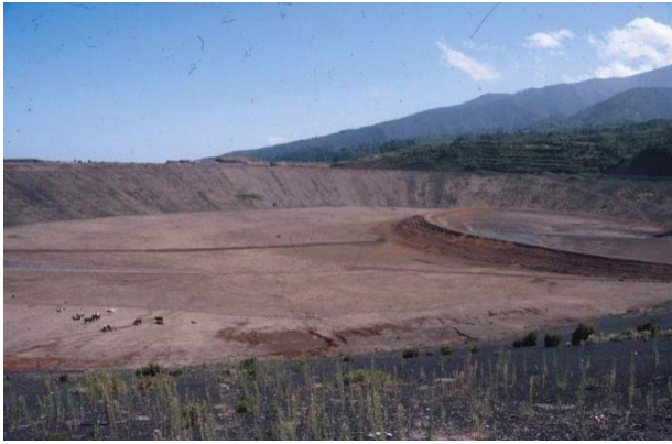
Figure 1. Barlovento, initial waterproofing carried out in 1976 with compacted volcanic clay
