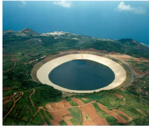
Figure 2. Barlovento, waterproofing with PVC-P geomembrane
